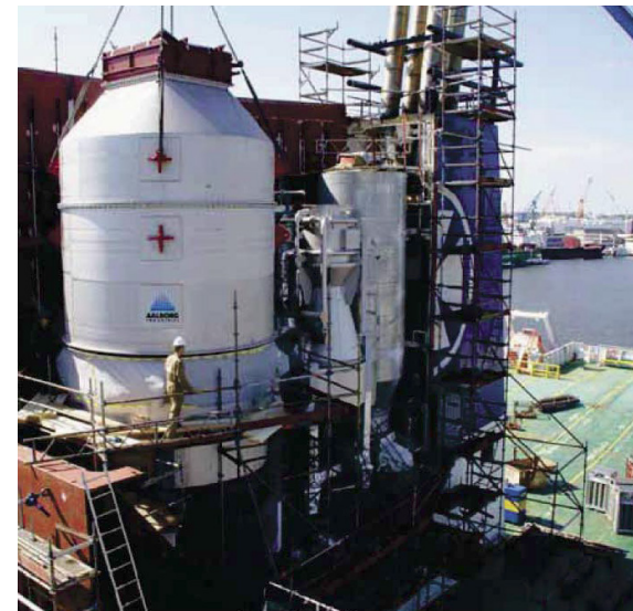
Pilot scrubber installation on DFDS vessel
